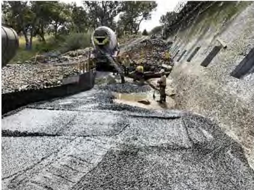
Photo Showing Toe Apron Slab Dental Concrete Installation
