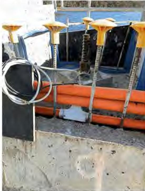
Photo Showing Anchor Monitoring Conduit and Anchor Connection
