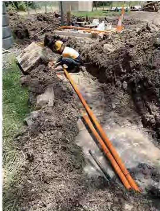
Photo of Monitoring Cable Conduit Being Installed to the Box
