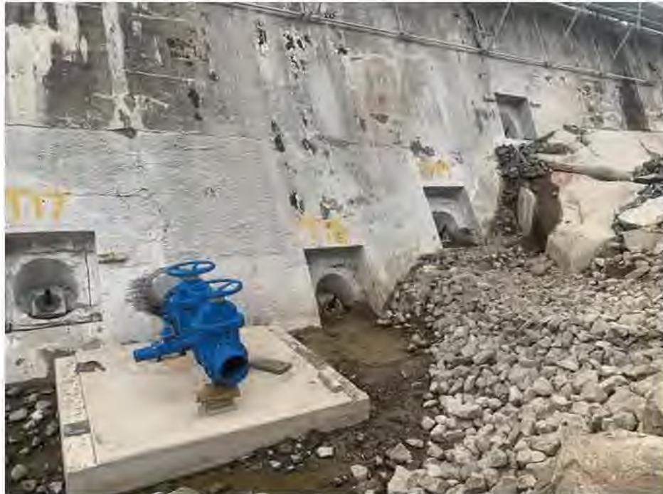
Photo Showing Installed D/S outlet Pipework and Valve
