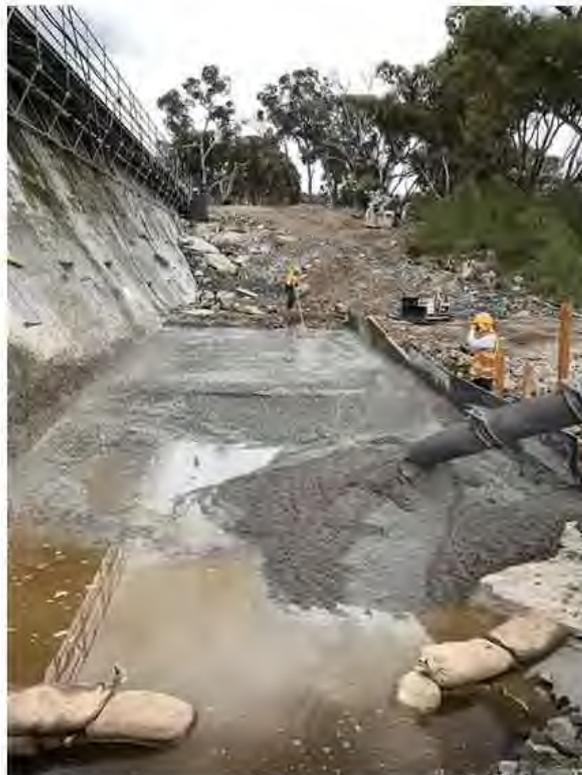
Photo Showing Toe Erosion Protection Slab Dental Concrete Pour Area
