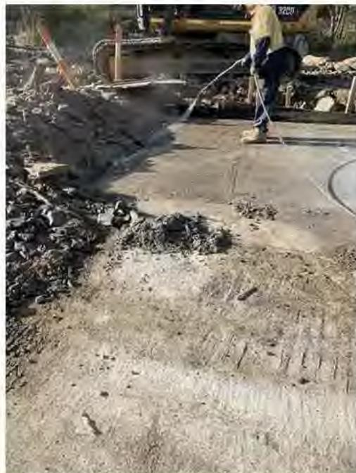
Photo Showing Green Cutting Toe Apron Dental Concrete
