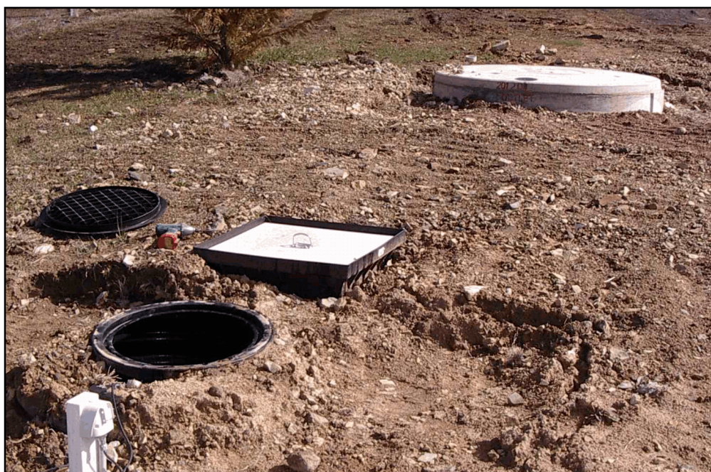
Figure D8: Septic tank flows into a filter tank, then a pump-well
