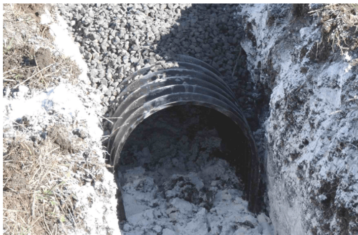
Figure D14: Lime spreading in trench
