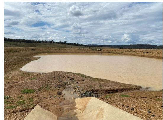
Photograph 5: Sediment Basin Inlet
